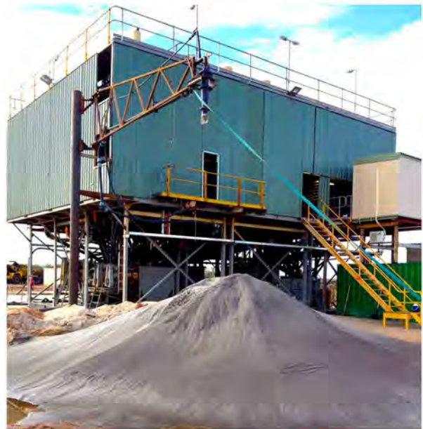
Rebuilt - the new concentrator plant 2012
